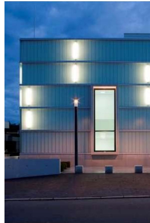
**Ventilated façade (cladding) with back illumination (neon lights)**
